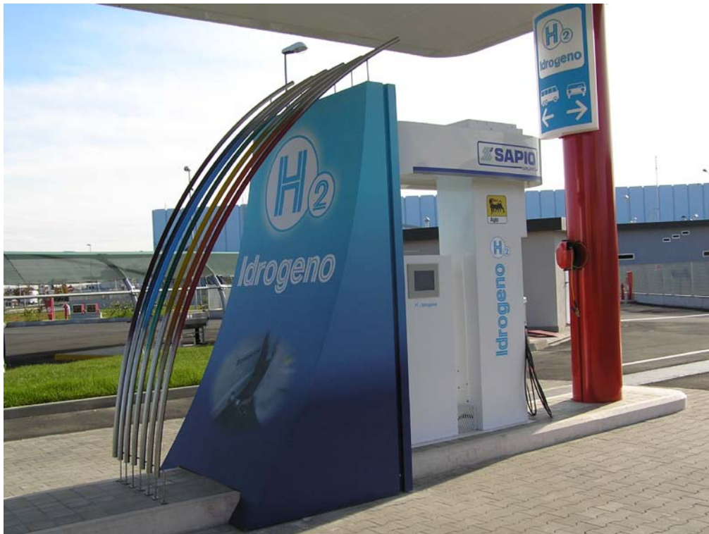
Fig.2: Hydrogen dispensers at the Mantova station
